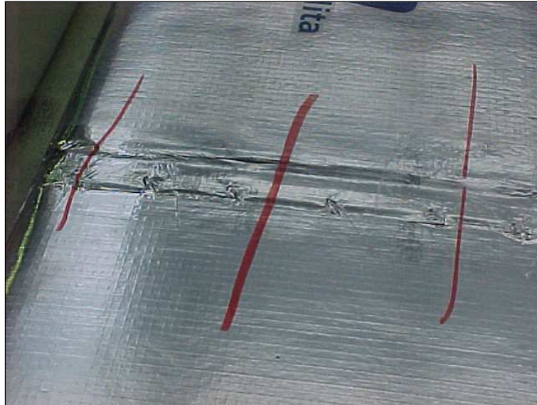
View of the peripheral joint after the test (P5858 sample)
